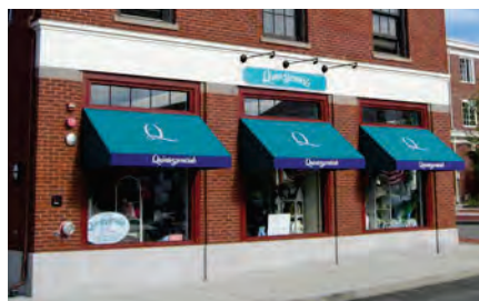
Vertical window proportions allow a traditional structural system with short spans and vertical piers to carry imposed loads to the ground.
